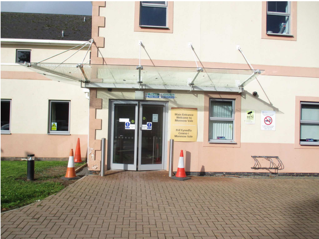
Photo 27 Level entrance/ automatic entrance doors.
