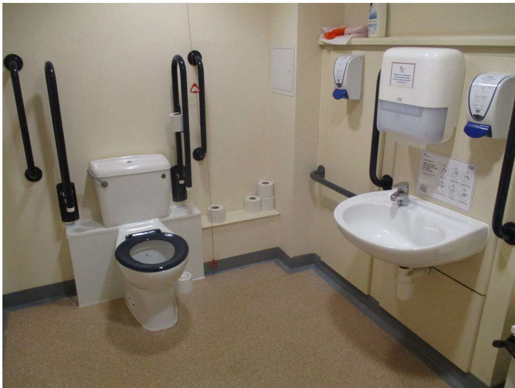
Photo 25 Peninsular layout accessible WC facility.
